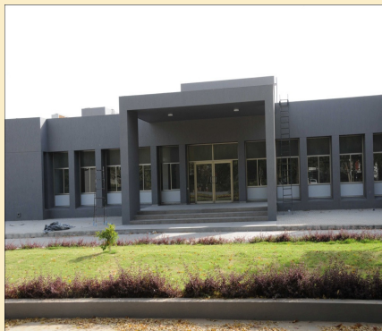
SEOC Building at Gandhinagar
